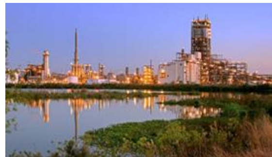
Polk Power Station Tampa Electric's Integrated Gasification Combined Cycle Power Plant (source: Tampa Electric)
